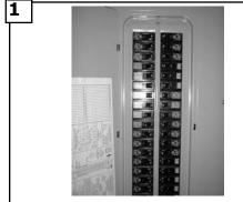
Before you begin installing the fan, Switch power off at Service panel and lock service disconnecting means to prevent power from being switched on accidentally. When the service disconnecting means cannot be locked, securely fasten a prominent warning device, such as a tag, to the service panel.
